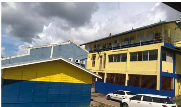
Part of the school building 1
