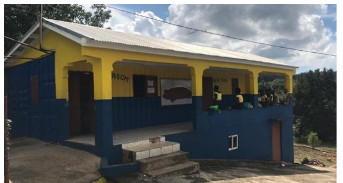
Part of the school building 2
