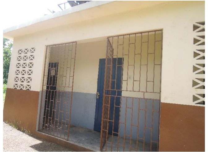
The bathroom had been closed but thanks to renovation, it can be used now.
