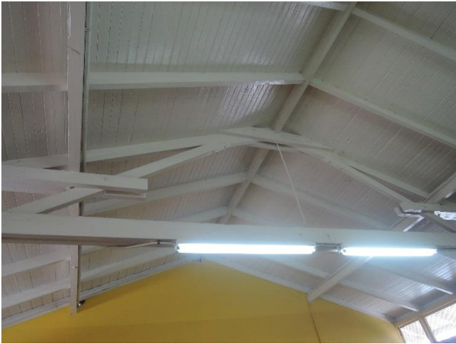
The room got new ceiling and electrical wiring updates.
