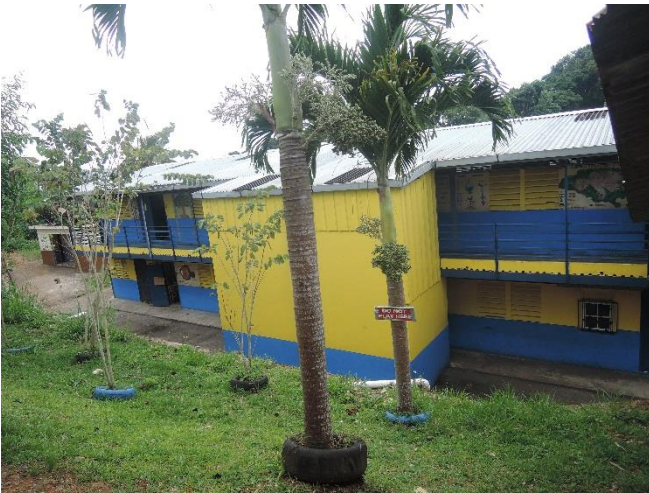
The building got painted, new doors and handrail through the funds.
