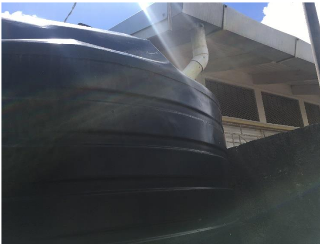
The gutter, pipe and water tank to catch, store and supply rain water
