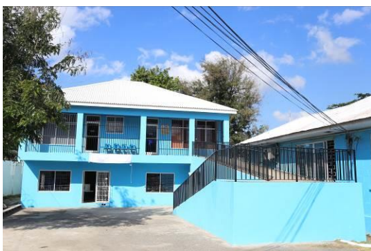
Newly constructed Top floor of the JSB Vision Centre funded by the Grant of Japan's GGP Programme.
